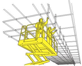
Figure 70: Scaffolders using a MEWP to erect a suspended scaffold.
