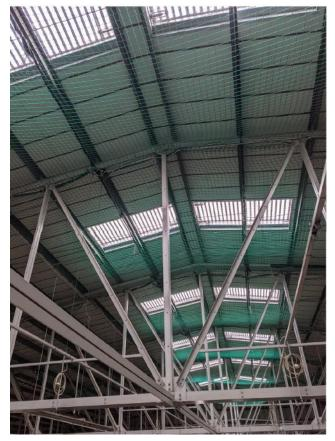
Figure 9: Example of protective measures for fragile surfaces with safety netting rigged below the roof surface. Source: FASET.
