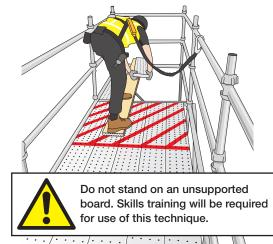
Figure 22: Example of an assembly aid to place and remove decking.
