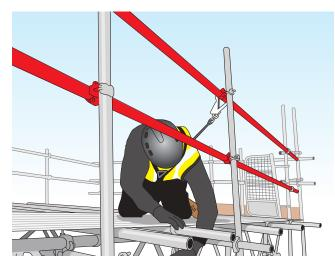
Figure 89: Shows perimeter edge protection to a traditional temporary roof.
