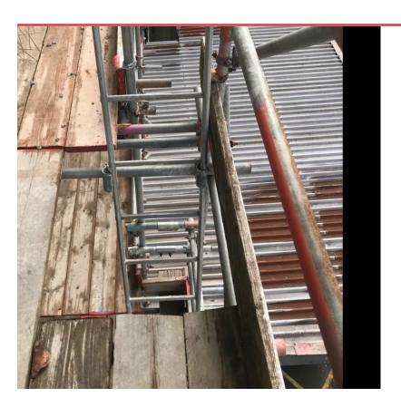
There is a Trap Door missing on the Working Lift that needs to be replaced in order for prevent falls from height and objects falling from height
