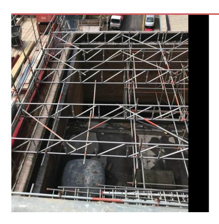
There are sufficient beams and ties on the scaffold on the South Elevation in order to meet the requirements of the Design and TG20:13
