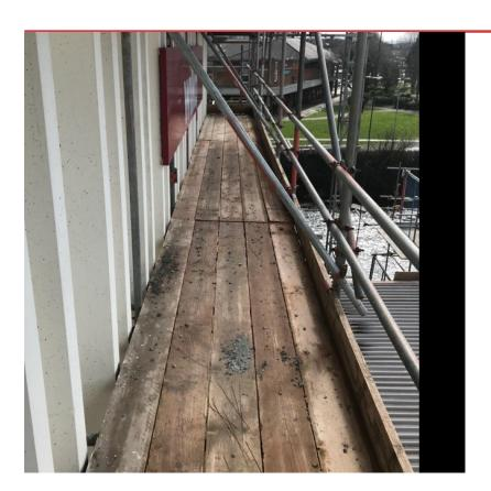
The Working Lifts were free from debris and waste materials on the Elevation nearest to the Rubbish Chutes
