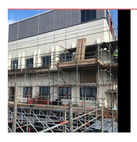
Scaffold materials need to be removed from Working Lifts in order to create greater access, as illustrated, Working Lifts have been removed from the scaffold in order to meet the ongoing requirements of the project.
