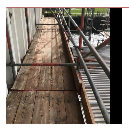
The Working Lifts were clear of waste and debris and the Housekeeping was of optimum condition but the scaffold materials need to be removed prior to next use
